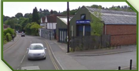
Site prior to demolition
